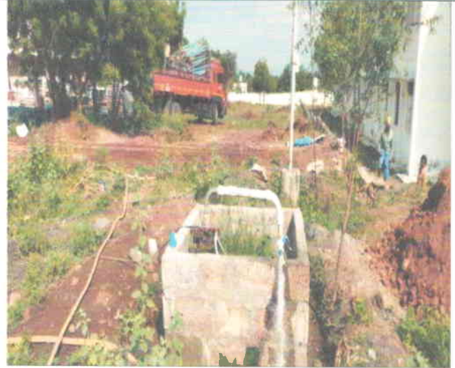
WATER IS POURING INTO THE TANK FOR THE CONSERVATION
