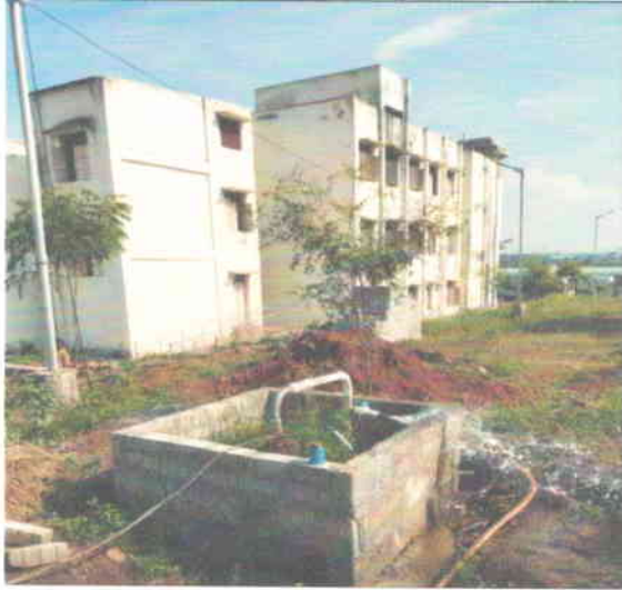
WATER CONSERVATION TANK BACKSIDE THE MAIN BUILDING
